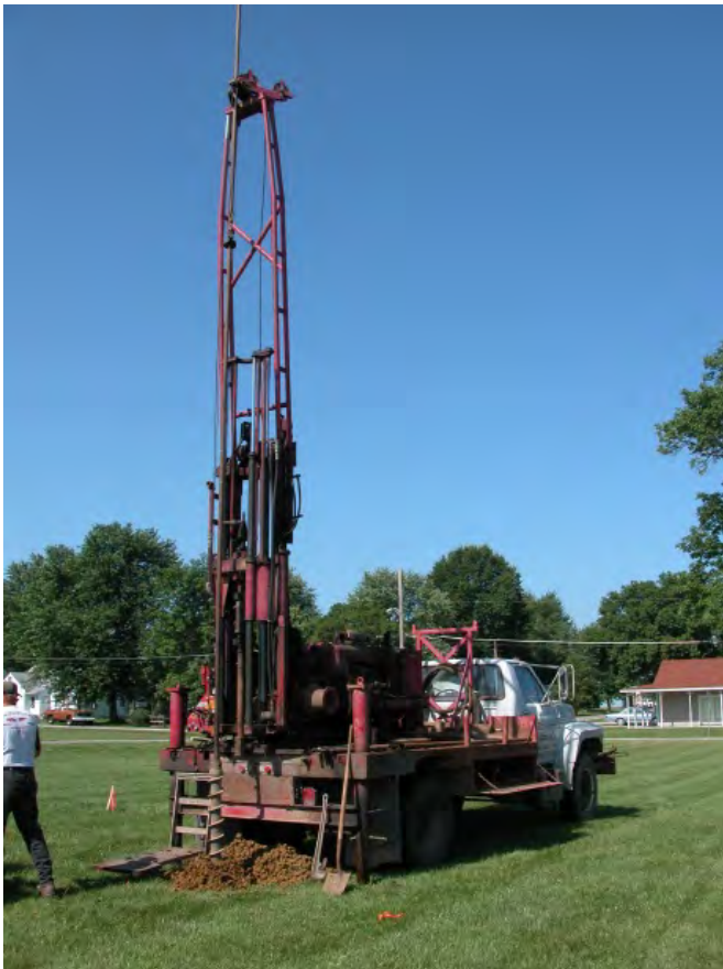
AUGER DRILLING OPERATION FIGURE 2-7
