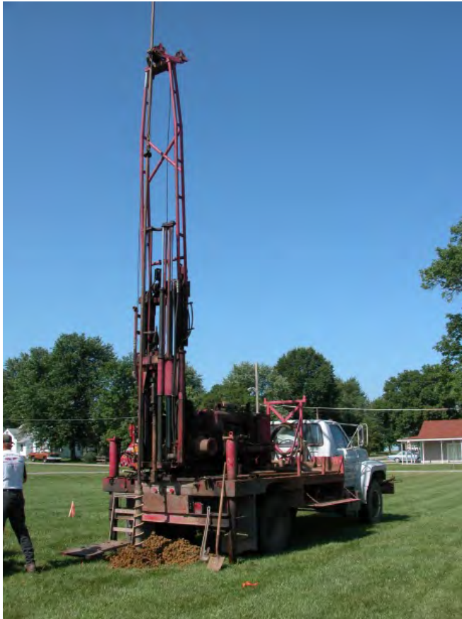
Auger Drilling Operation Figure 2-7
