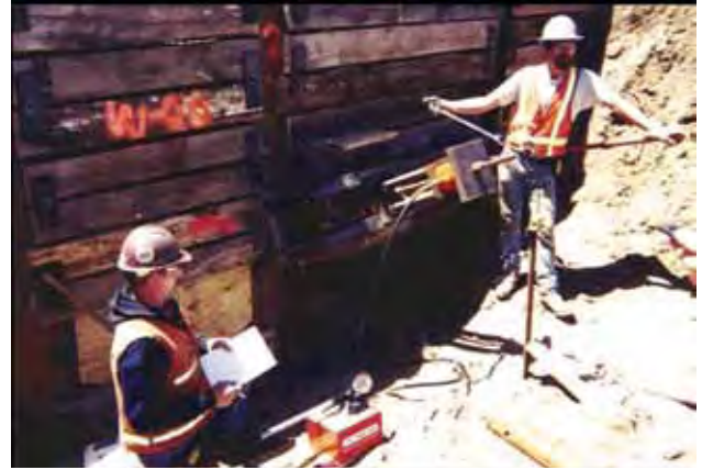
Anchor Tension Load Test in Minneapolis, MN Figure B-2
