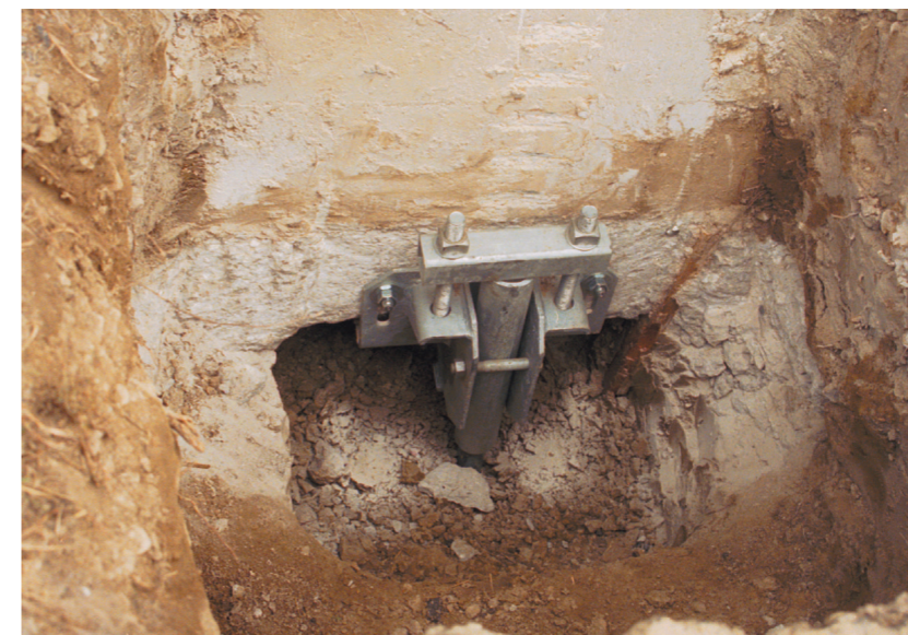
Completed helical pile and bracket
