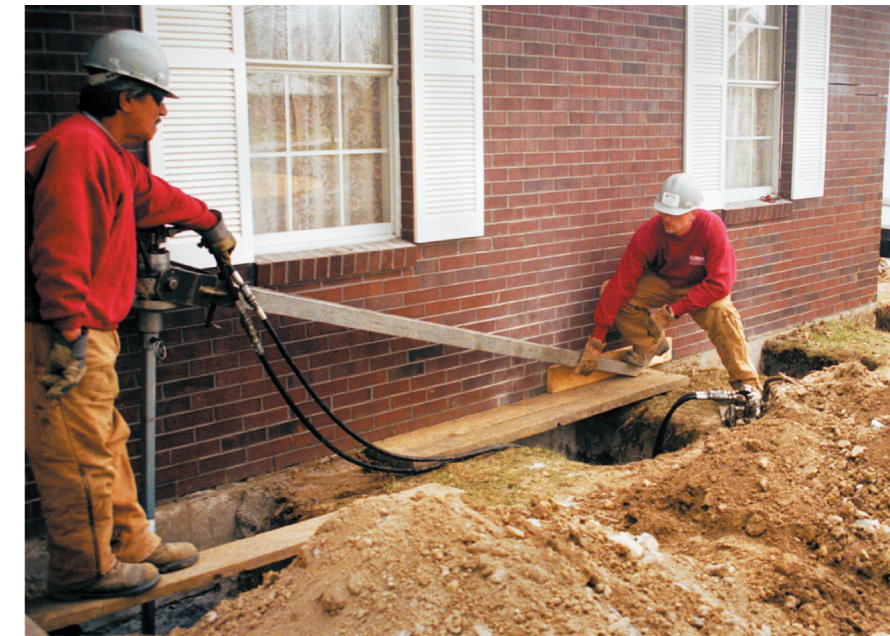
Helical pile installation by hydraulic driver
