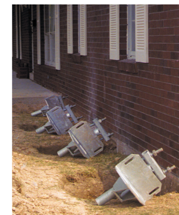
Helical pile shafts are cut off, then brackets are attached.
