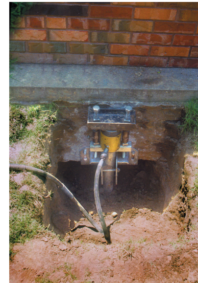
Hydraulic jack pushes down on helical pile shaft and up on foundation held in bracket. After jacking, nuts on top of T-pipe secure the load. Then, jack and plate above are removed to complete installation.
