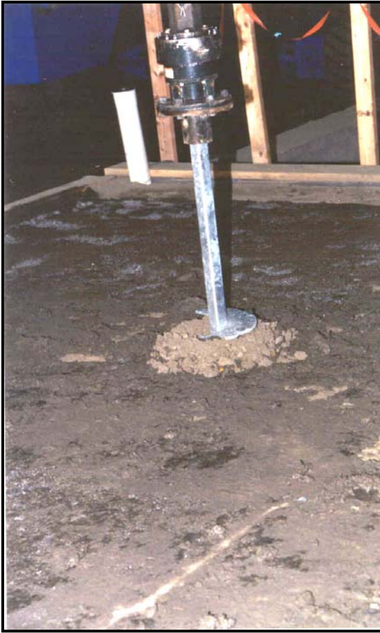
Figure 3.20 Pier Installation
