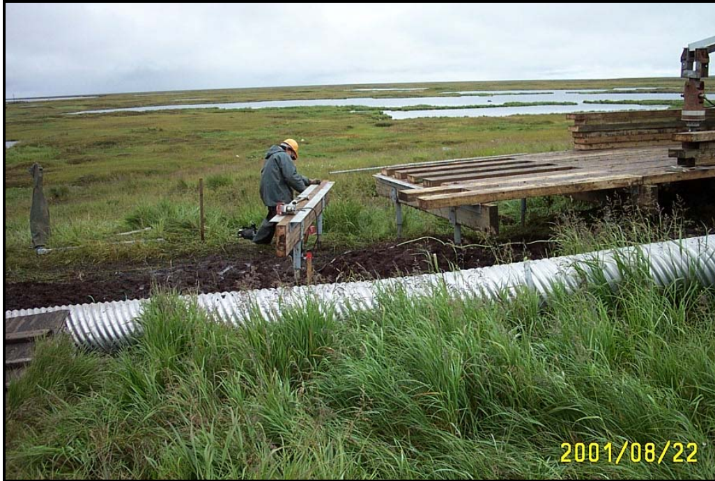
Figure 4.10 The Summer Installation of the Boardwalk in Chefnak. (VSW) The Power Head on the Skid Loader Used to Install the Piers can be seen at the Right.
