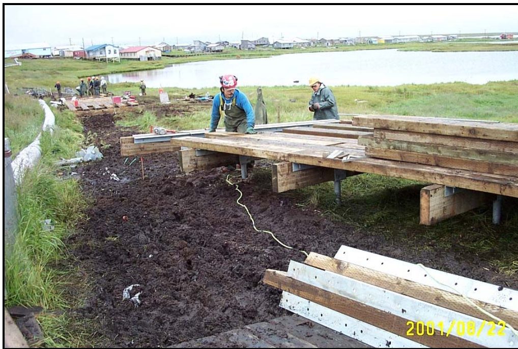
Figure 4.11 Installation of the Boardwalk in Chefnak (VSW)
