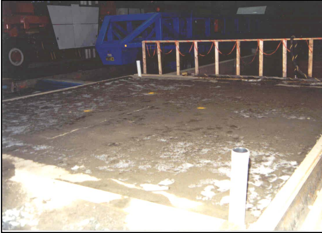
Figure 3.8 Frozen Test Cell Prior to Pier Installation (from South)
