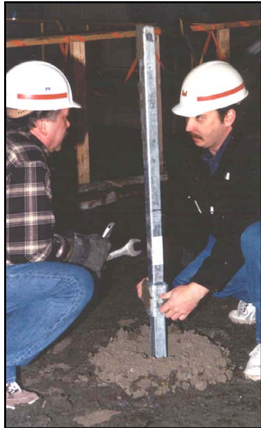
Figure 3.21. Pier Extension is Attached
