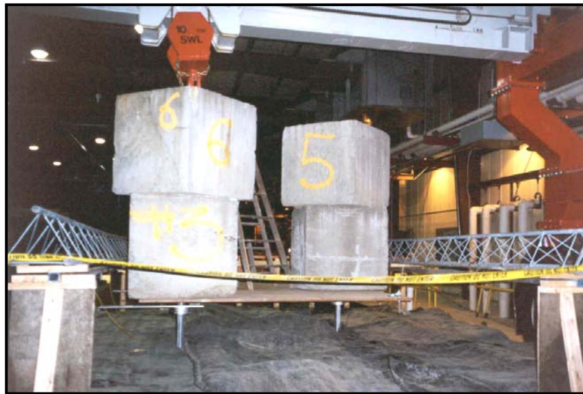
Figure 3.26 Loading Piers with Six Concrete Blocks
