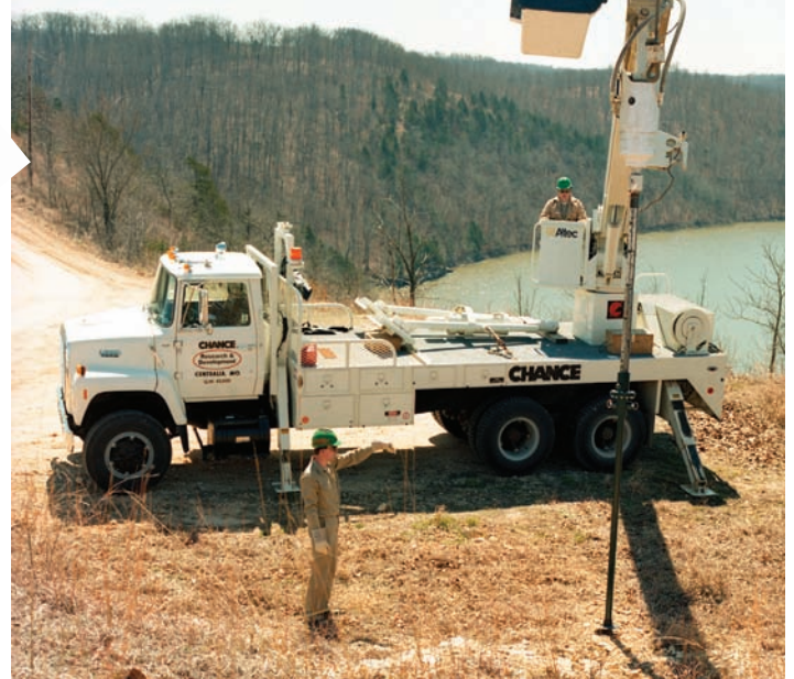
PISA® anchor installation takes about 5 minutes with two workers.
